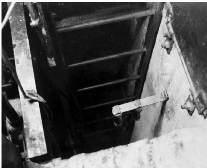
Boulder Canyon. View showing target used in optical plumbing observations attached to inset in NV wall of elevator shaft at El. 974.
