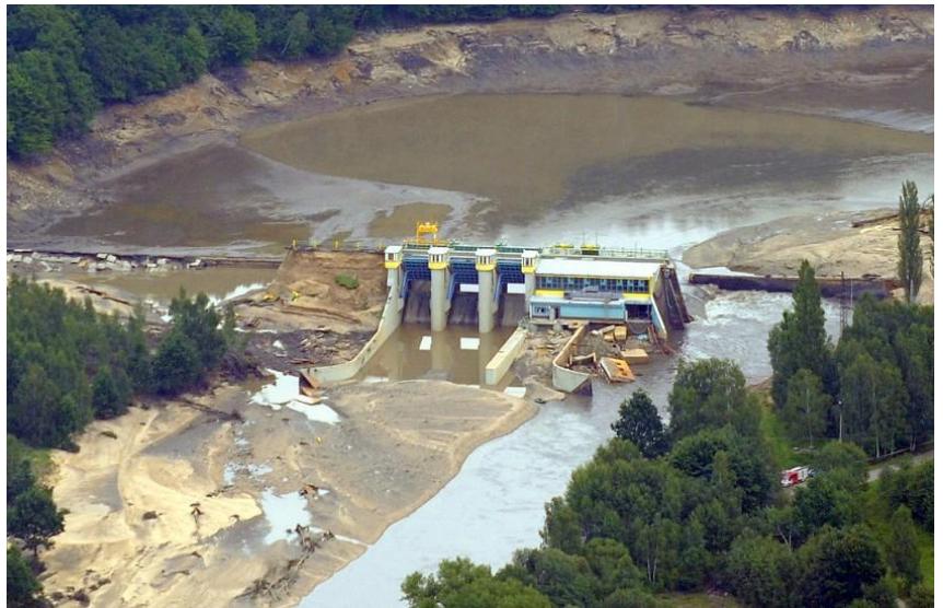
Witka dam, Poland, collapsed on August 7, 2010
