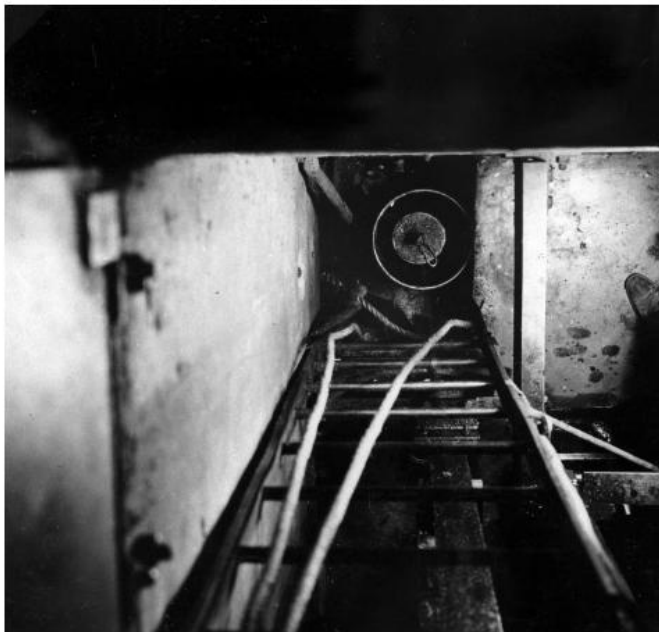
Caption: Boulder Canyon. Plumb bob, suspended in can of oil at bottom Shaft, used in plumbing observations.
